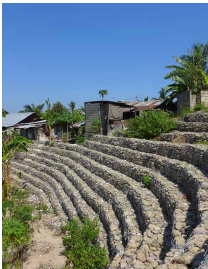
Figure 9: (Left) The destruction of this sea wall indicates the failure of this strategy in protecting coastal settlements. Mangroves, cultivated with the cooperation of the coastal community, offer an environmentally sound alternative. (Right) Retaining walls are one of the effective methods of overcoming the problem of landslides in Kupang's hilly topography.
