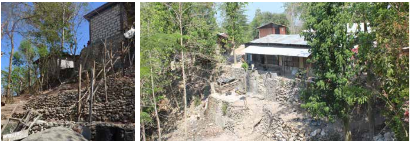
Figure 28. The steep sides of the ravines in Bello are quickly becoming inhabited as households look for available land and living opportunities in the area. There have already been numerous landslides here that have resulted in injury and death; this will only worsen with more heavy rain and the construction of precarious housing on steep slopes.
