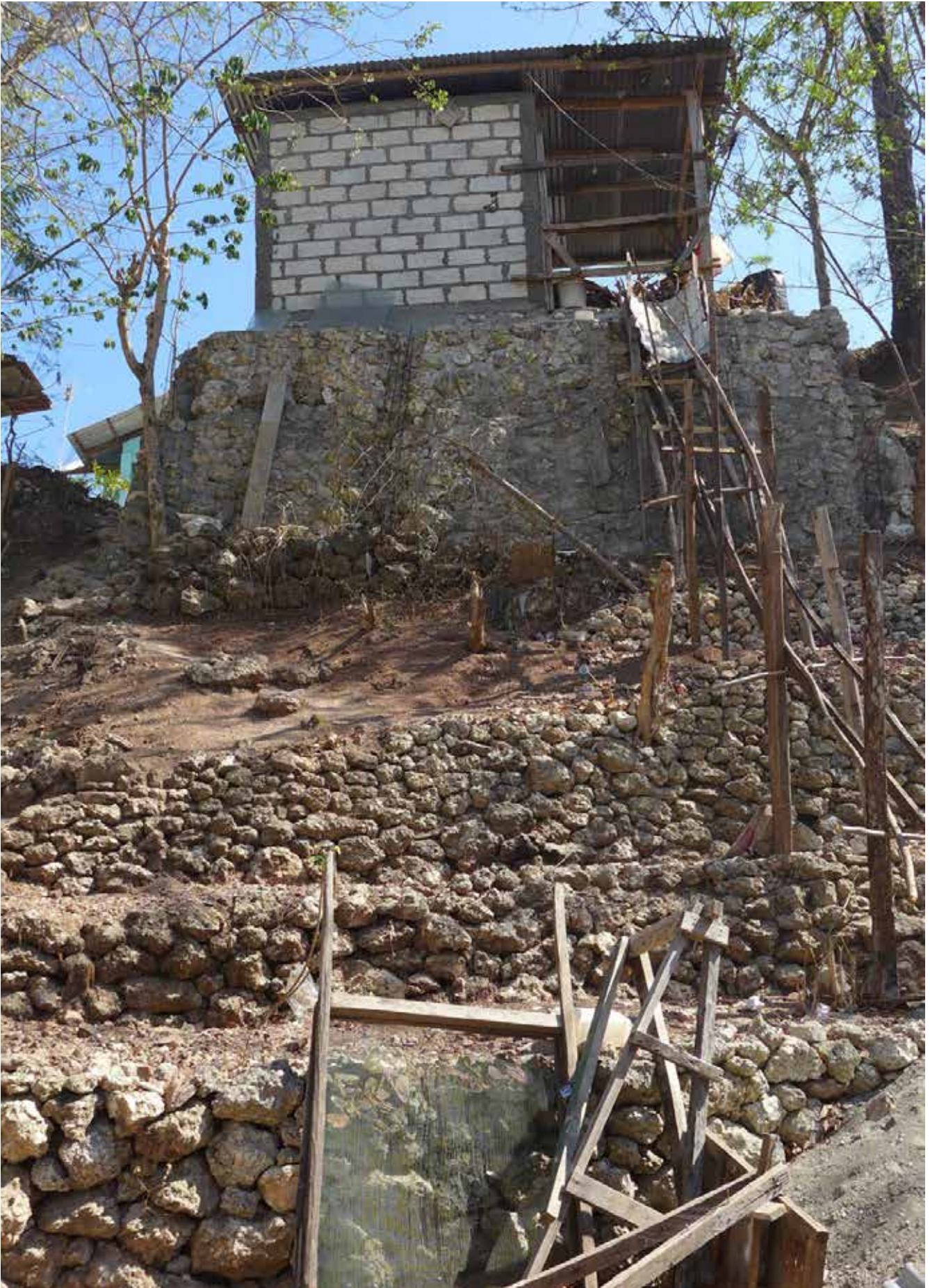
Figure 19. Households living along ravines, as in the case of those in Bello, are exposed to the risk of landslides during the rainy season, usually in January and February. As more and more people move to these areas they often cut down trees and vegetation promoting erosion. Falling rocks and material can cause damage to homes and injury people -- making these vulnerable areas.
